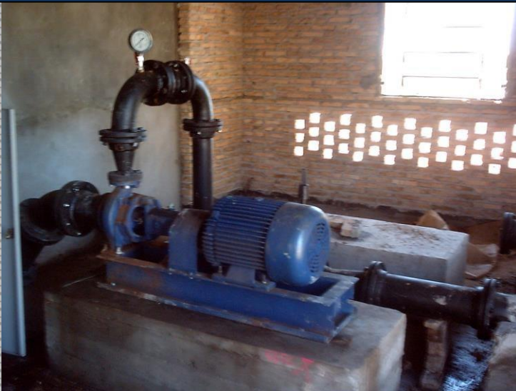
Pumps of 30 Hp of Tank Drive of 150 m3
