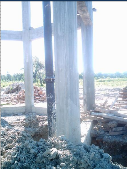
View of the 200-foot drop pipe of the 150 m3 Elevated Tank
